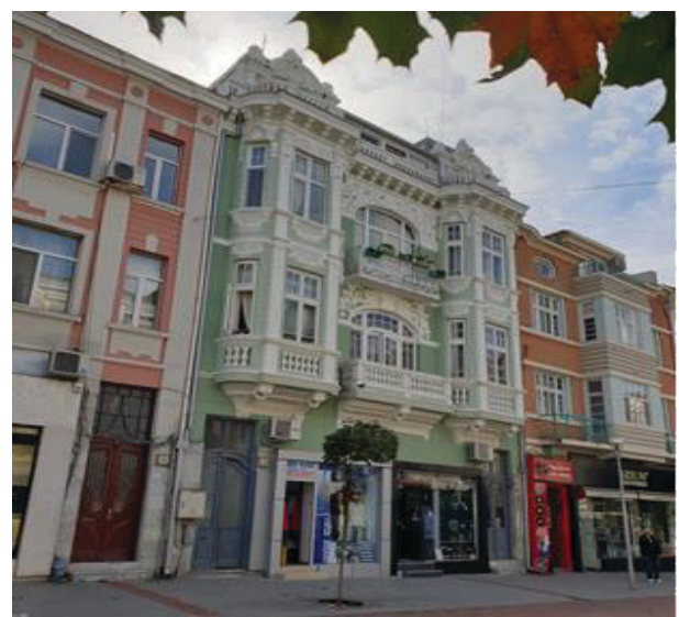
Fig. 17. The main façade of the building after restoration.
